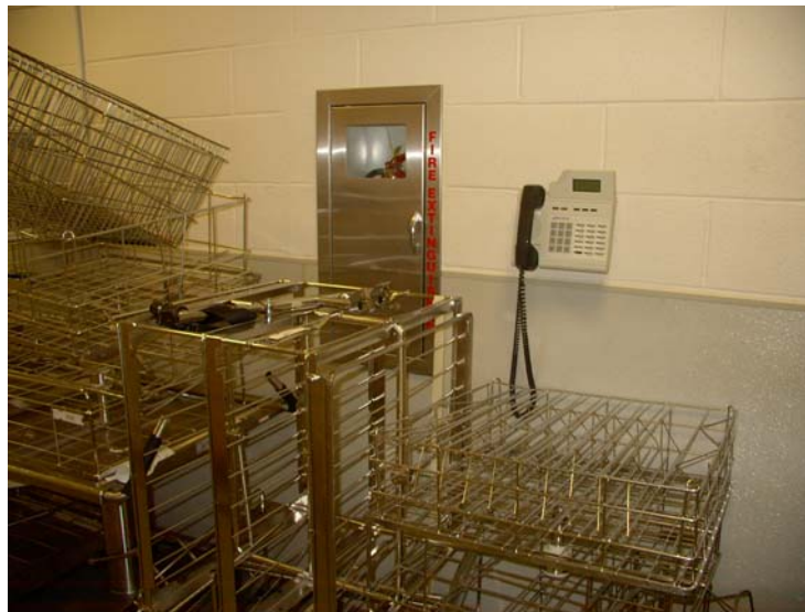
Too bad we can't reach the Fire Extinguisher
